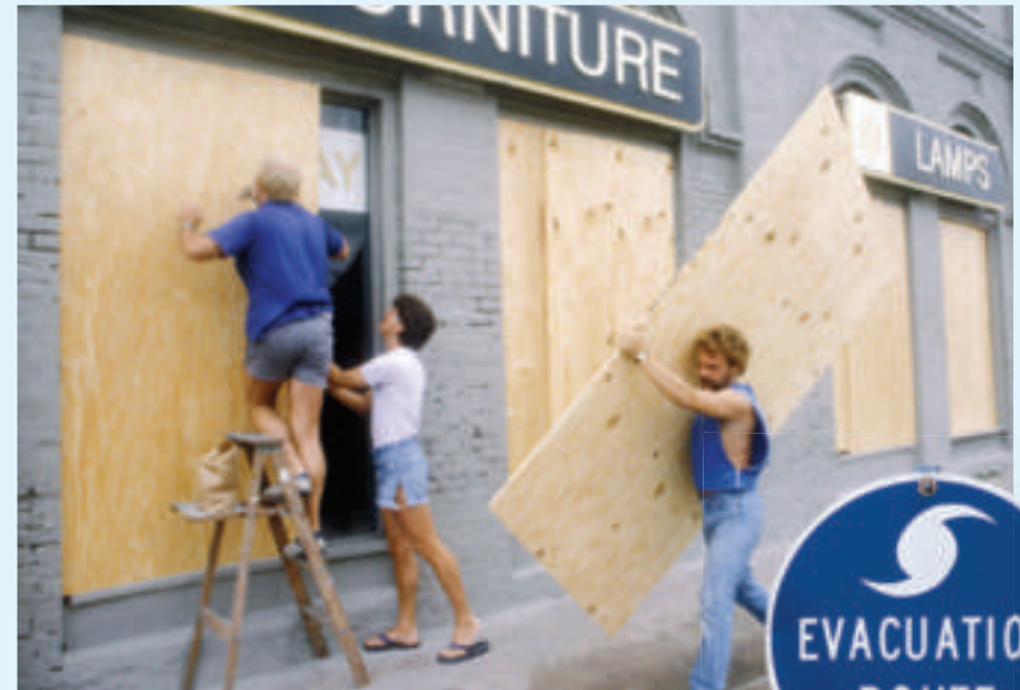
Windows should be boarded up before a hurricane to keep them from being smashed.
